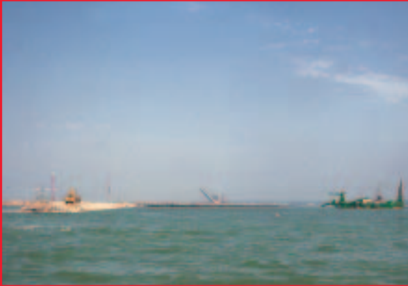
Cutter dredger VLAANDEREN XIX is extracting the gravel from the future swinging basin...
