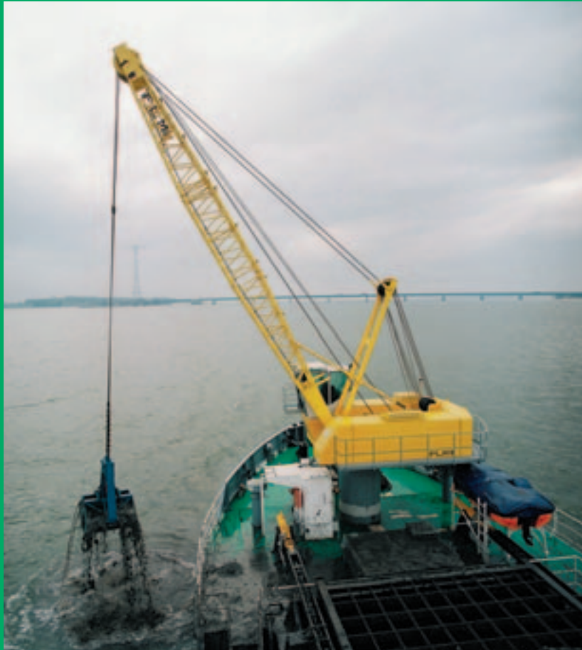
Grab crane during dredging trials
